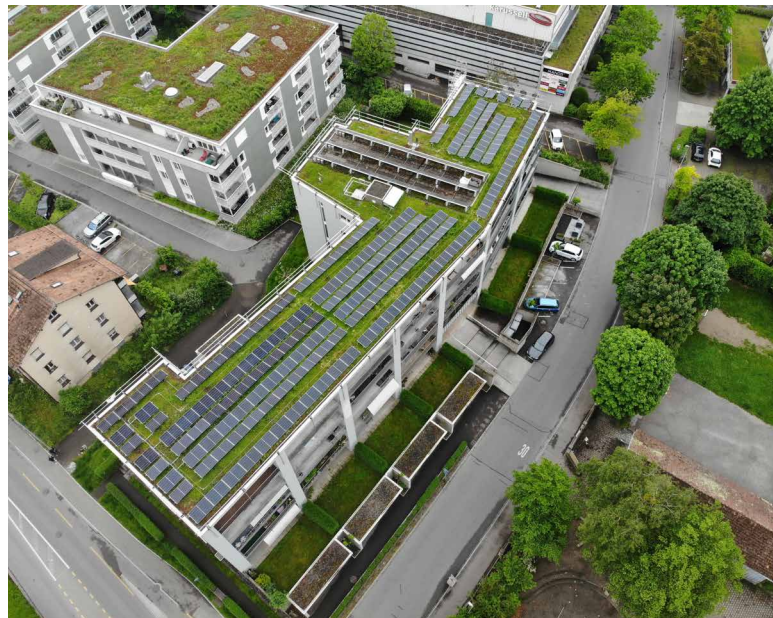
Photovoltaikanlage in Kreuzlingen
