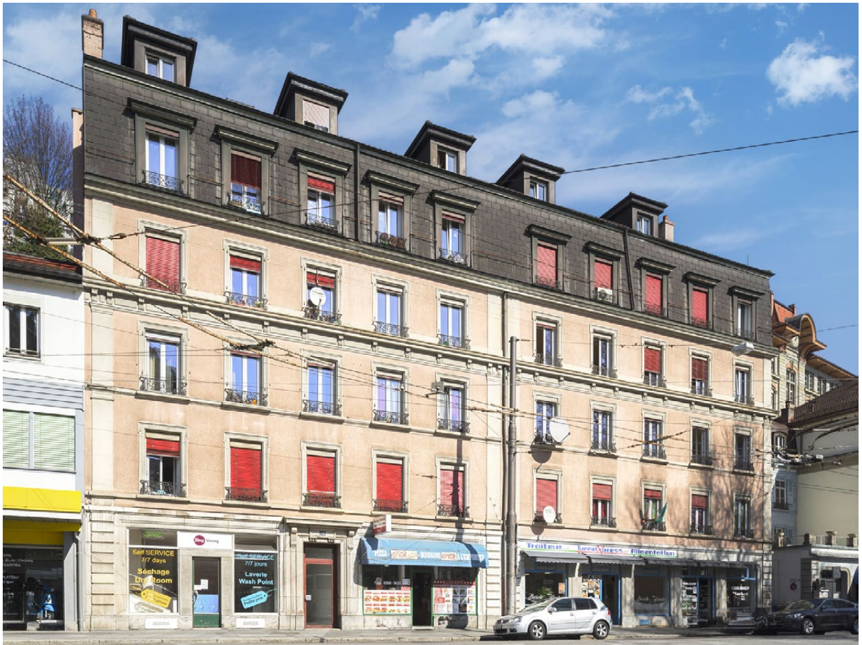
Tunnel 13–14, Lausanne (VD)
