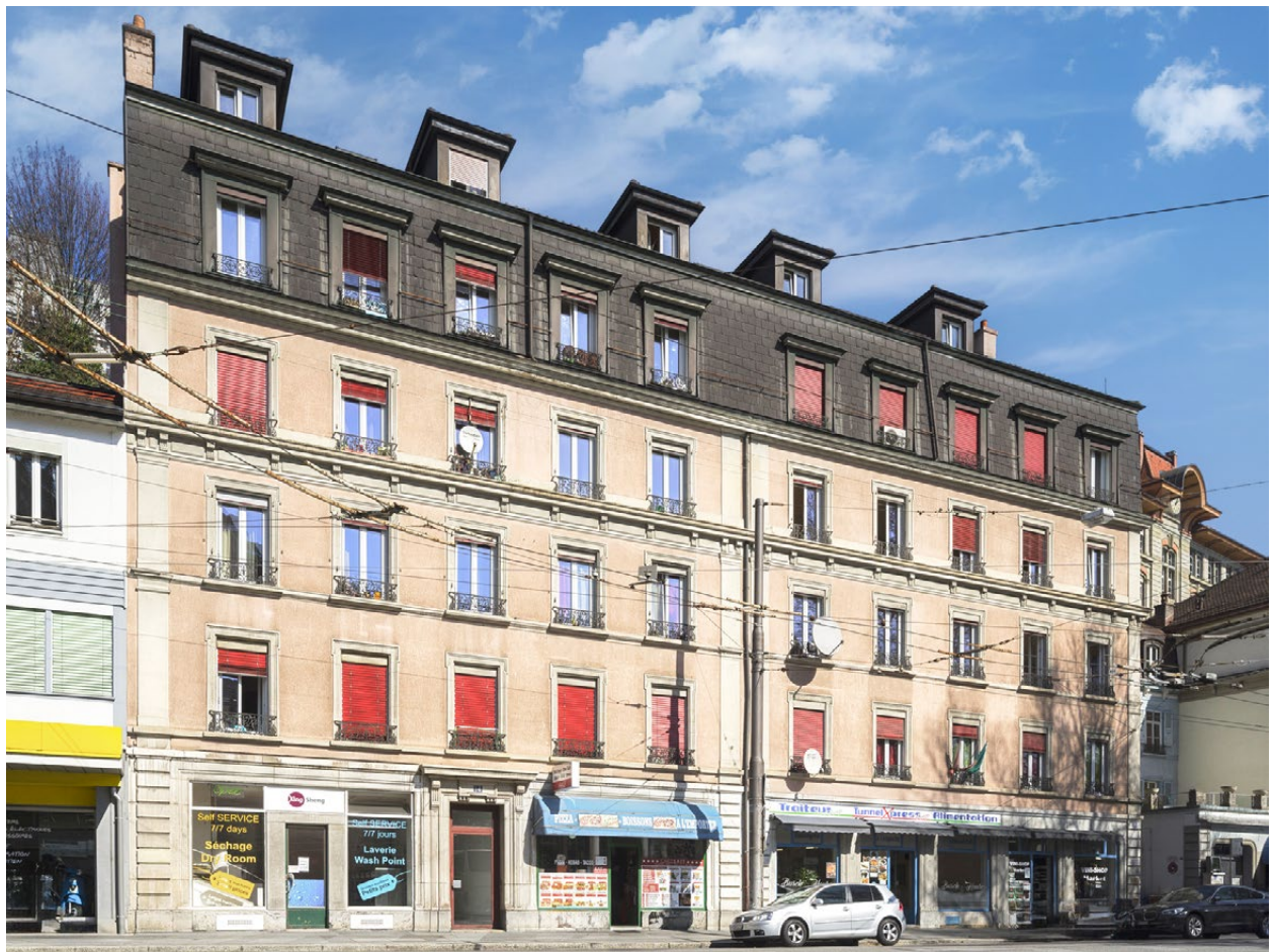
Tunnel 13–14, Lausanne (VD)
