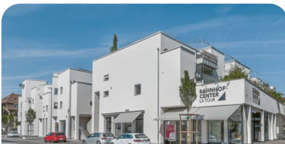
Lyss Bahnhofstrasse 7-13 / Bielstrasse 14
